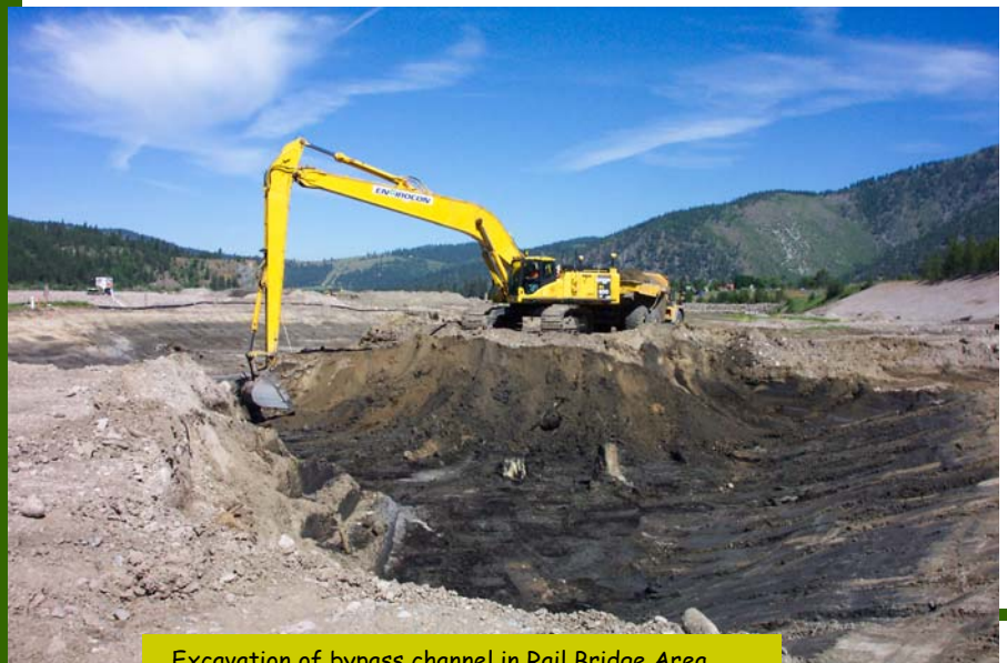
Excavation of bypass channel in Rail Bridge Area
